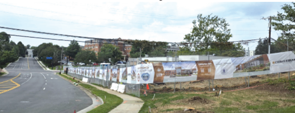
Willard-Sherwood redevelopment construction: early September 2026 (image TINP)
