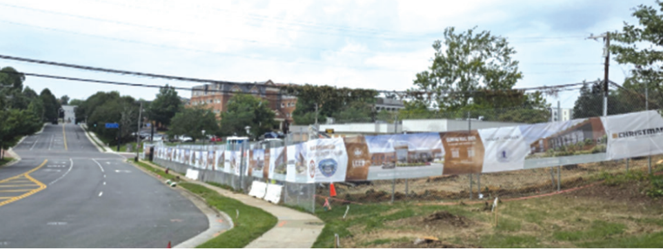
Willard-Sherwood redevelopment construction: early September 2026 (image TINP)
